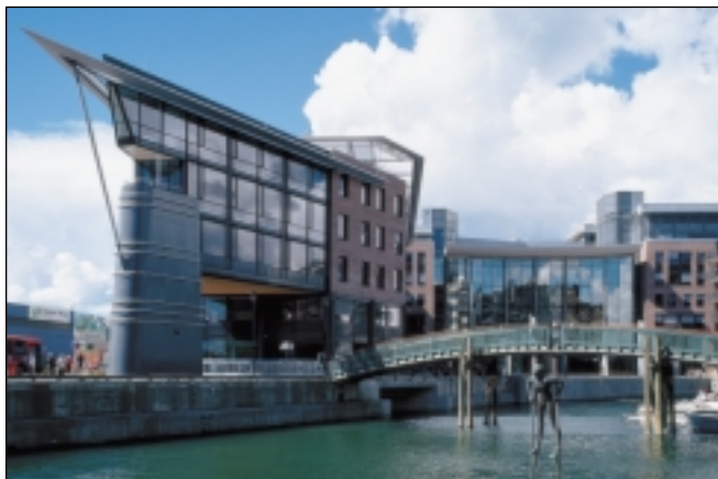
Storebrands head office at Filipstad Brygge in Oslo.
