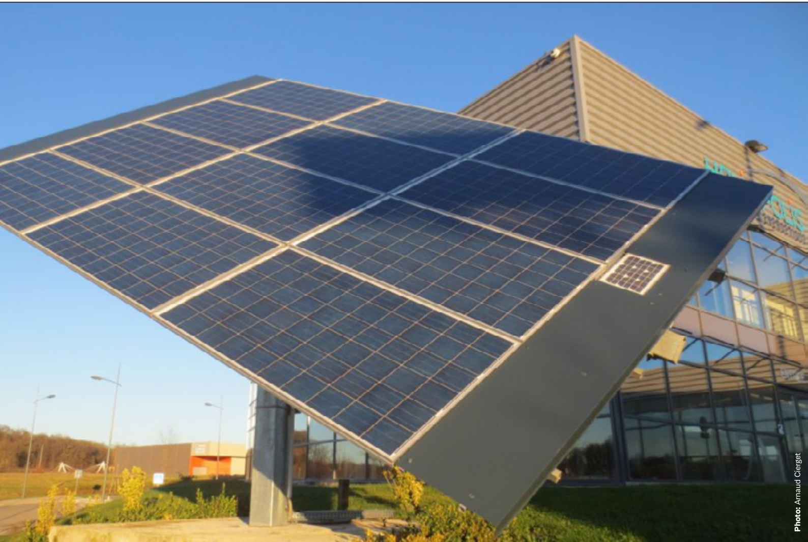
↑ Solar panels mounted on a tracking system.
